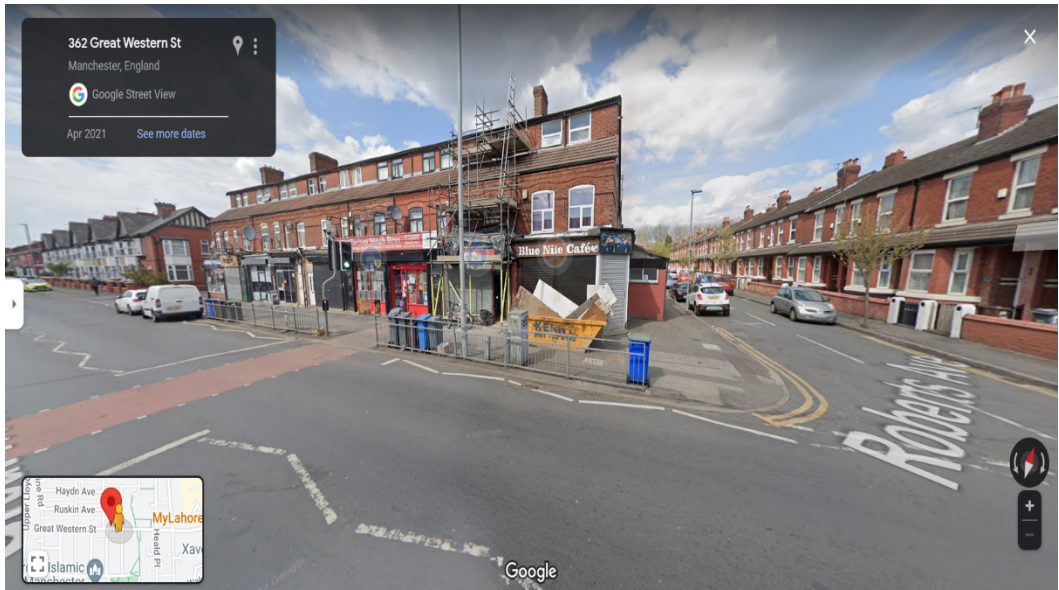
Google Image showing proximity to residential properties. (Scaffolding outside Admas Café location)
